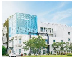
Waste treatment center
