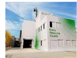
Waste solvent recycling plant
